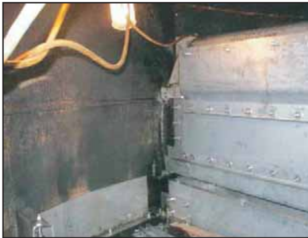
Figure 5 Flash box supported, using feed pipe and existing tower attachments
