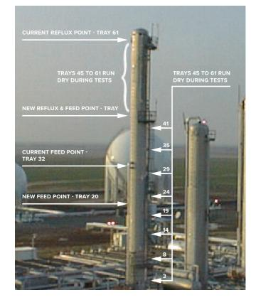
The empirical O'Connell correlation can be used to predict overall column efficiencies (Eoc) for ULTRA-FRAC trays. With this Test and Demonstration unit, we can confidently predict ULTRA-FRAC efficiencies.
