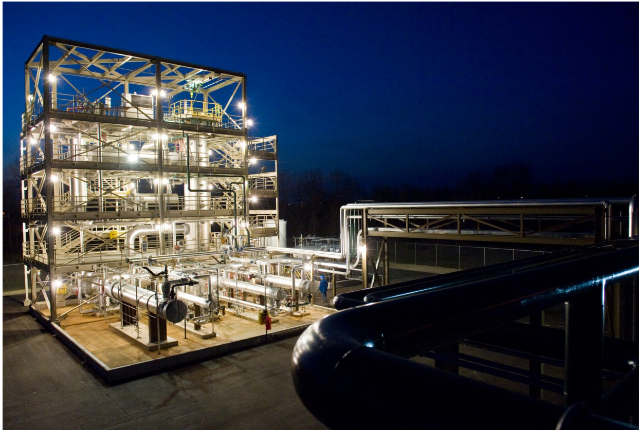
Koch-Glitsch 5.5 ft [1.7 m] diameter hydrocarbons distillation tower, Wichita, Kansas
